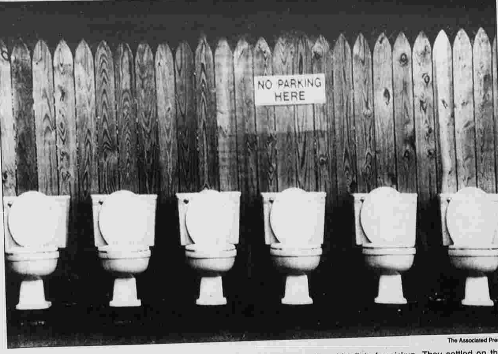
ALL IN A ROW — When a motel in Roanoke, Va., began renovating recently, workmen had to find a place to temporarily store the old toilets for pickup. They settled on the parking lot, right under the no parking sign.
